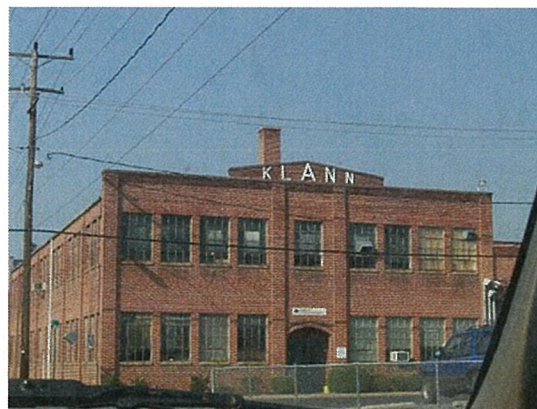
Example of Group F structure, the Klann Organ Company, located in Waynesboro, Virginia.
