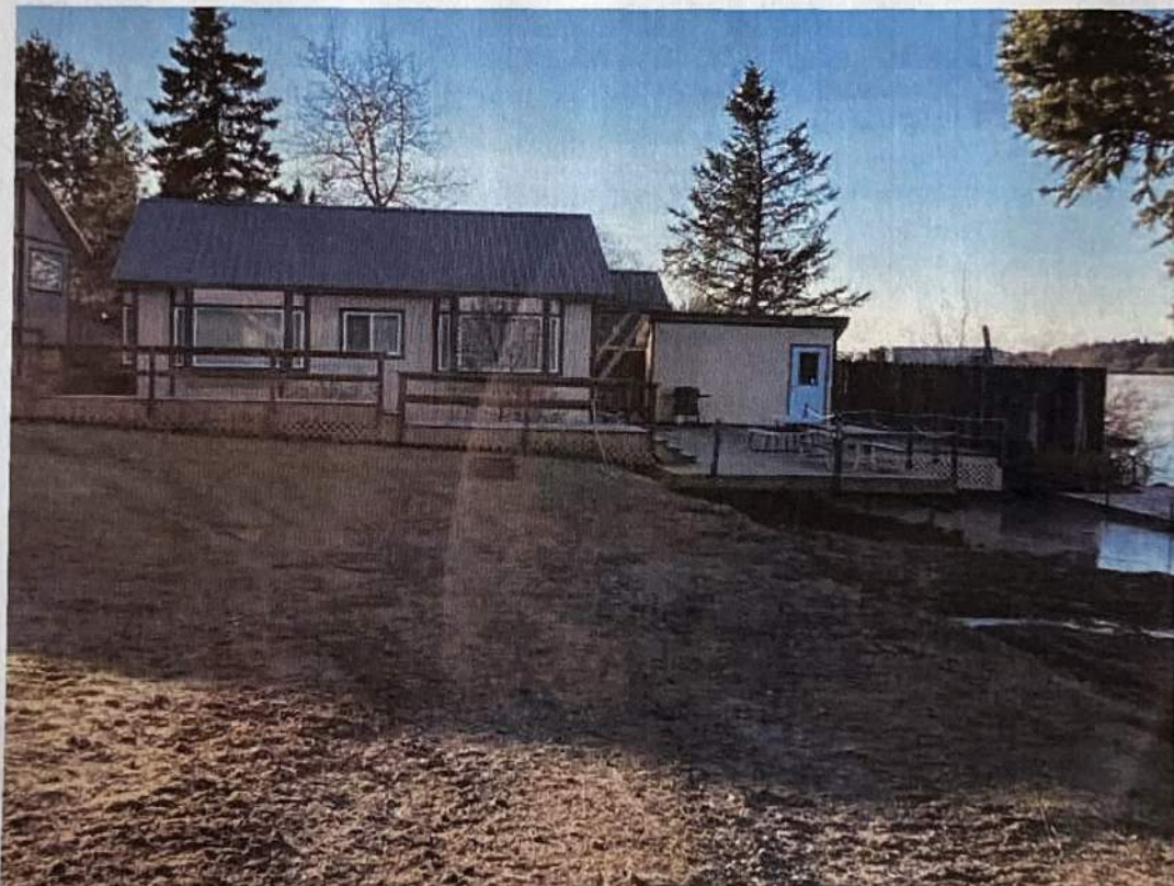
SHORELINE LOOKING SOUTHEAST AT EXISTING CABIN.
