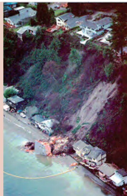
Landslide destroys home on Bainbridge Island, Washington, within seconds in 1997, killing four.
