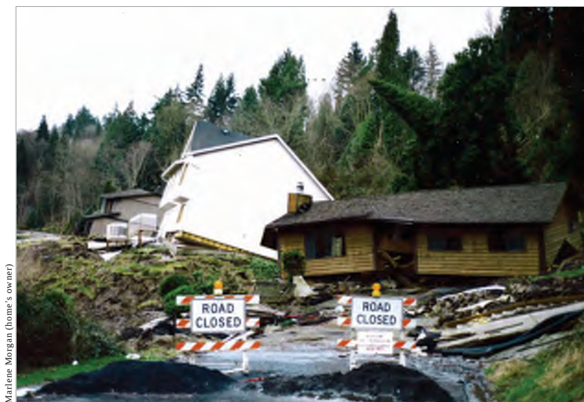
A house in Kelso, Washington, torn apart by the landslide in 1999.
