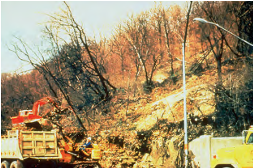
The image shows earthflow material being removed by a highway crew along the Columbia Parkway. Hamilton County, in the metropolitan Cincinnati area, experienced an average annual economic loss from landslides of $5.80 per person (1975 dollars) between 1973 and 1978, the highest calculated per capita loss of any municipality in the United States.
