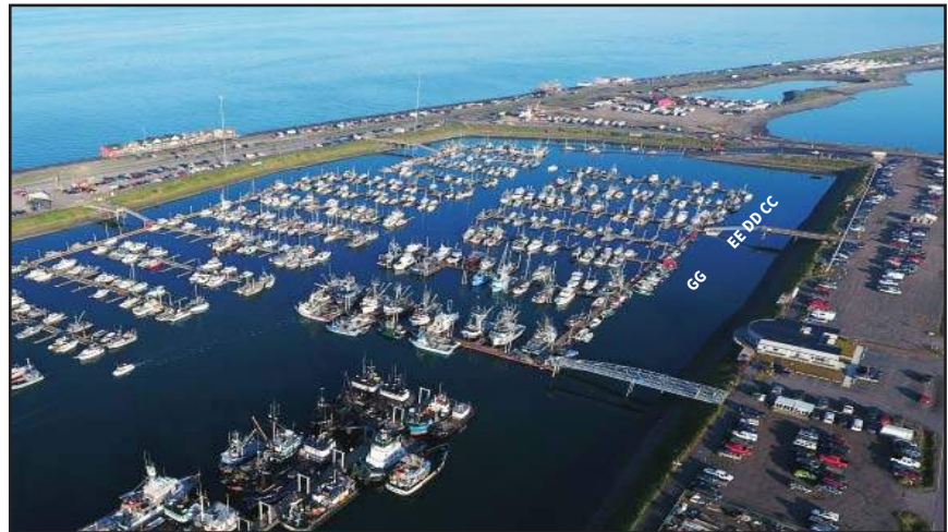
System 4 ramps to be replaced next.
