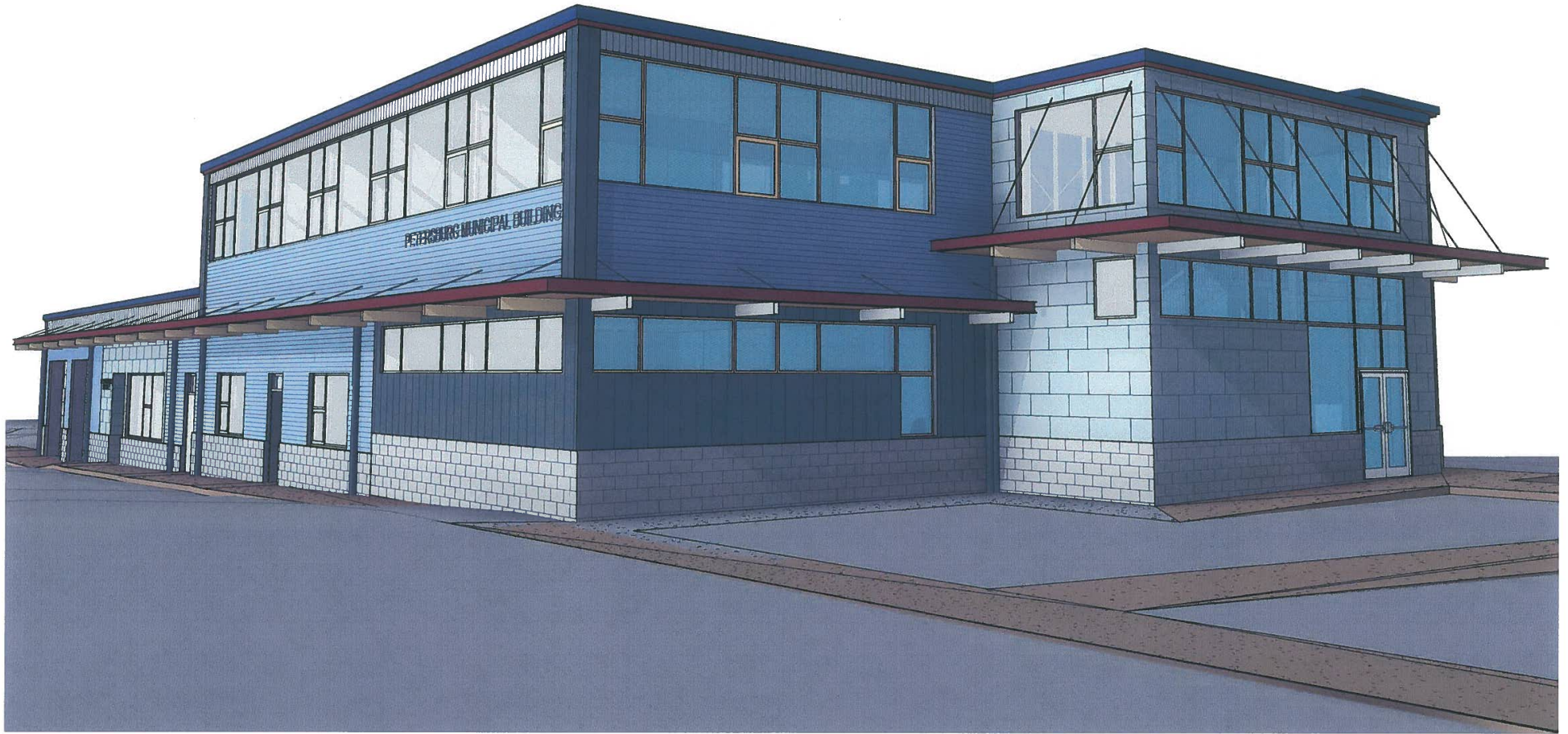
Petersburg Municipal Building Renovation NE Corner
