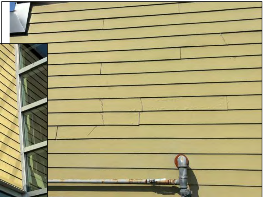
Examples of damaged and broken siding on the library
