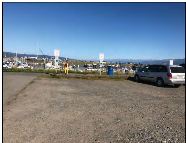
While inaccessibility issues in these Port & Harbor parking spaces have been remedied, it provides an example of spaces needing to be paved with an even path of travel.
